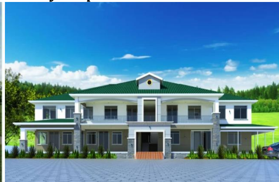
Dental school under construction For training of public health dental officers starting 2025
